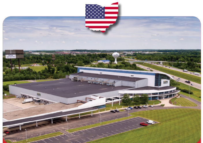
Modula Plant - Franklin, Ohio
