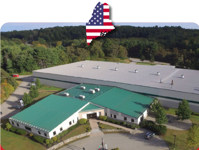
Modula Headquarters and Plant - Lewiston, Maine
